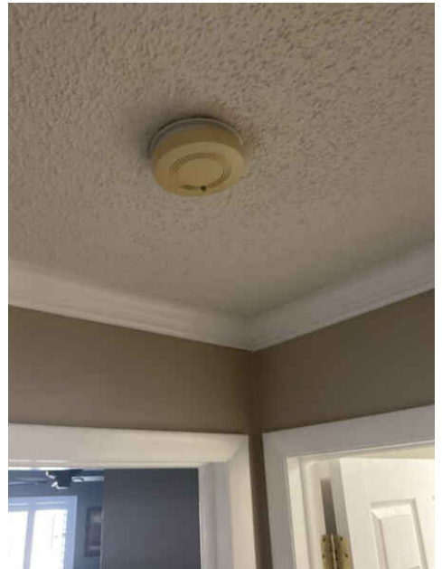
In hallway by laundry room
